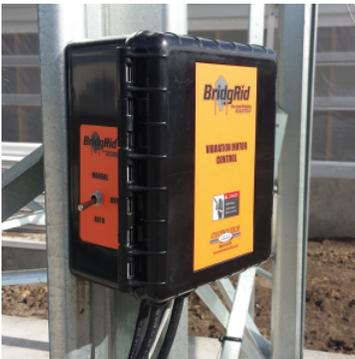
BridgRid electronics provide 24/7 automation. Sensors monitor the feed in the tube when the auger is rotating and agitation occurs only as necessary.
